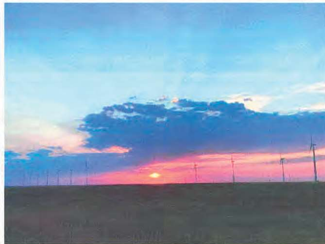
Windfarm, Lamar, Prowers County, Southeastern Plains
