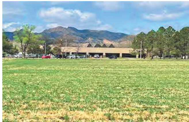
The Abby Events Center, Canon City; Fremont County
