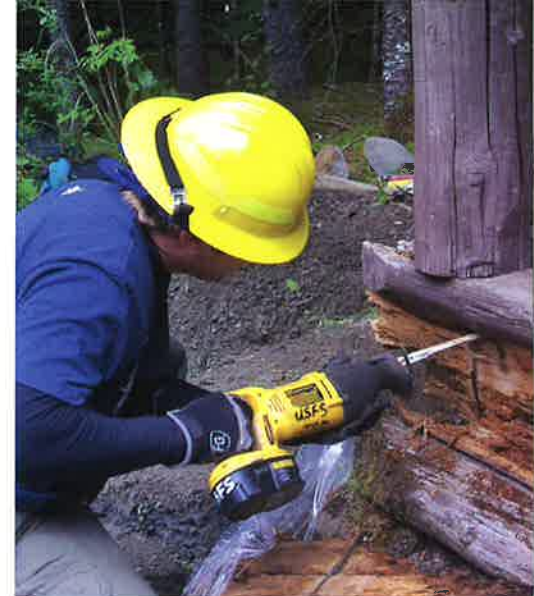
Restoration work at Cobble Shelter, AK
