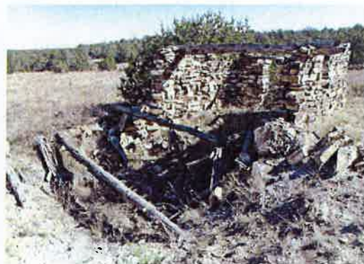
5LA.11778 Dugout with later addition
