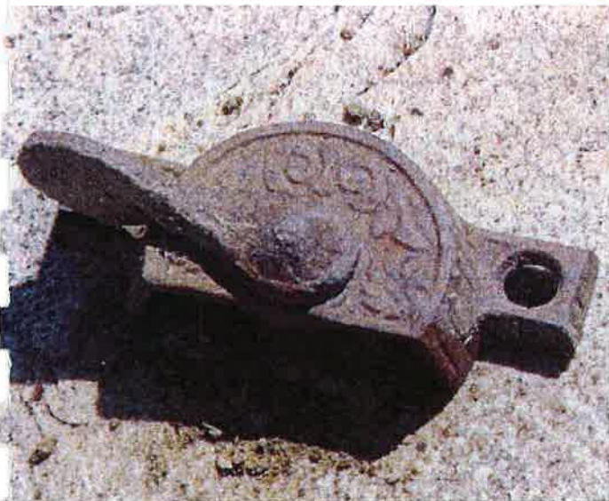
Embossed decorative cast iron sash window lock, ca. late 19th century
