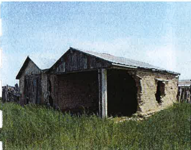
5LA.11897 Adobe block construction
