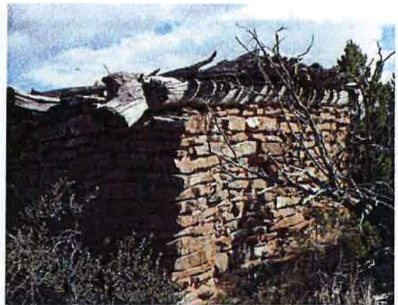
5LA.11761 Viga and latia roof construction
