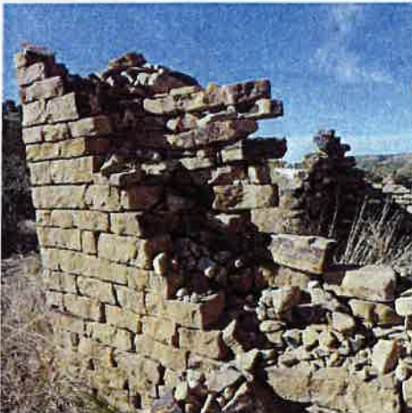
5OT.1105 Double stone wall construction
