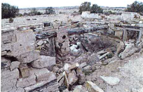
5LA.11895 Dugout constructed with stone and a roof of railroad ties
