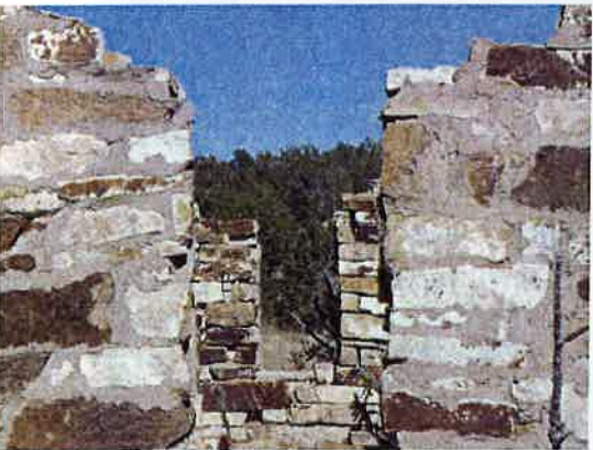
5LA.11809 the exterior of this dwelling has been repointed with concrete but the original adobe mortar is still visible on the interior
