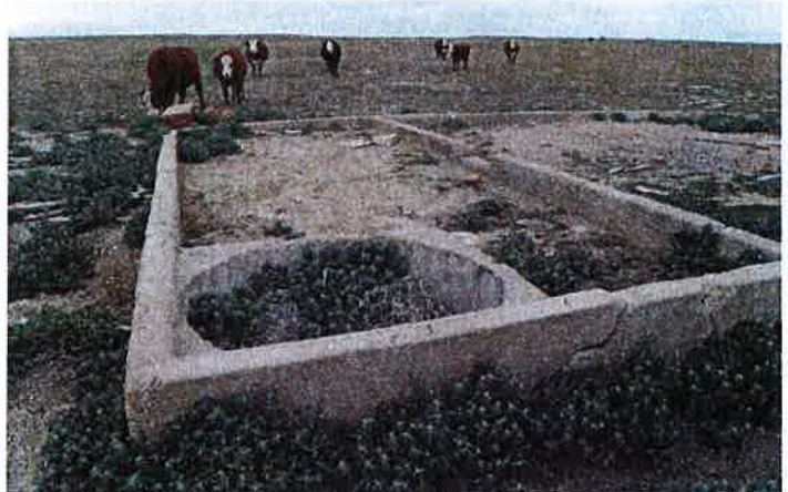
5OT.1112 House foundation with corner cistern
