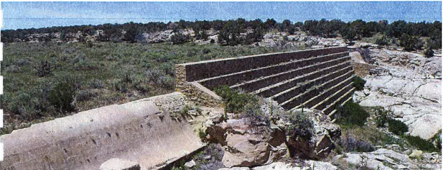
LA.11600. The AT&SF constructed this dam across Timpas Creek near Thatcher in 1895 in order to collect water for use by its steam engines. The locomotives' boilers required a large amount of water and water stations were located every five to twenty miles. The water from the dam was piped to an elevated water tank located adjacent to the railroad tracks.
