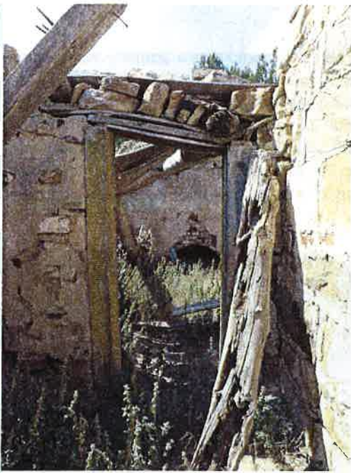
5LA.11635 Interior of dwelling
