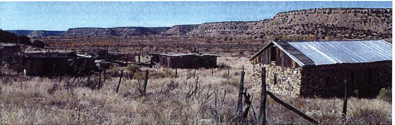
5LA.11736. The architecture of the Vidal Villareal homestead reflects largely New Mexican building traditions, including the use adobe bricks, vigas and latias in roof construction, and jacal construction. Villareal also incorporated his buildings into the natural landscape, such as incorporating a large rock outcropping into a chicken house. The ability to fully utilize the natural features is seen often in Hispanic homesteads. Coming from a region with a similar climate and landscape, New Mexican homesteaders were better equipped to deal with the challenges of life in the semi-arid Purgatoire River Region.
