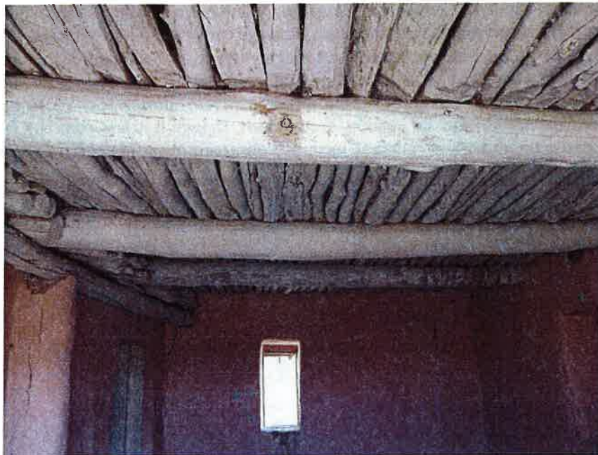
5LA.11736 Interior view of viga and latia roof construction
