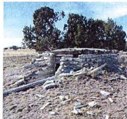
5LA.11895 Dugout constructed with stone and a roof of railroad ties
