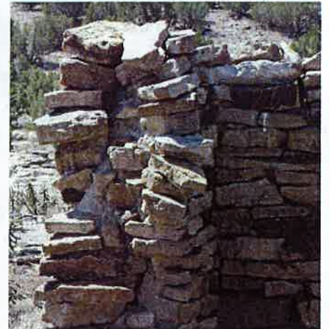
5LA.11676 Double stone wall construction
