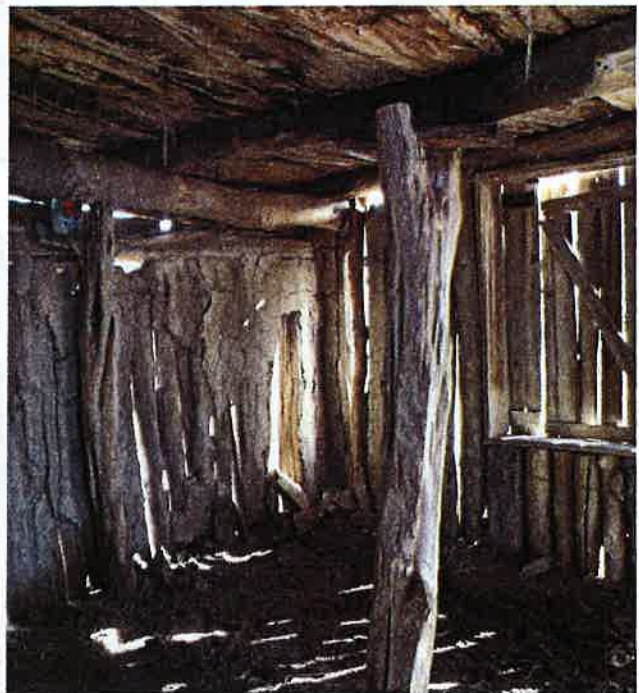
5LA.11736 Interior of jacal structure
