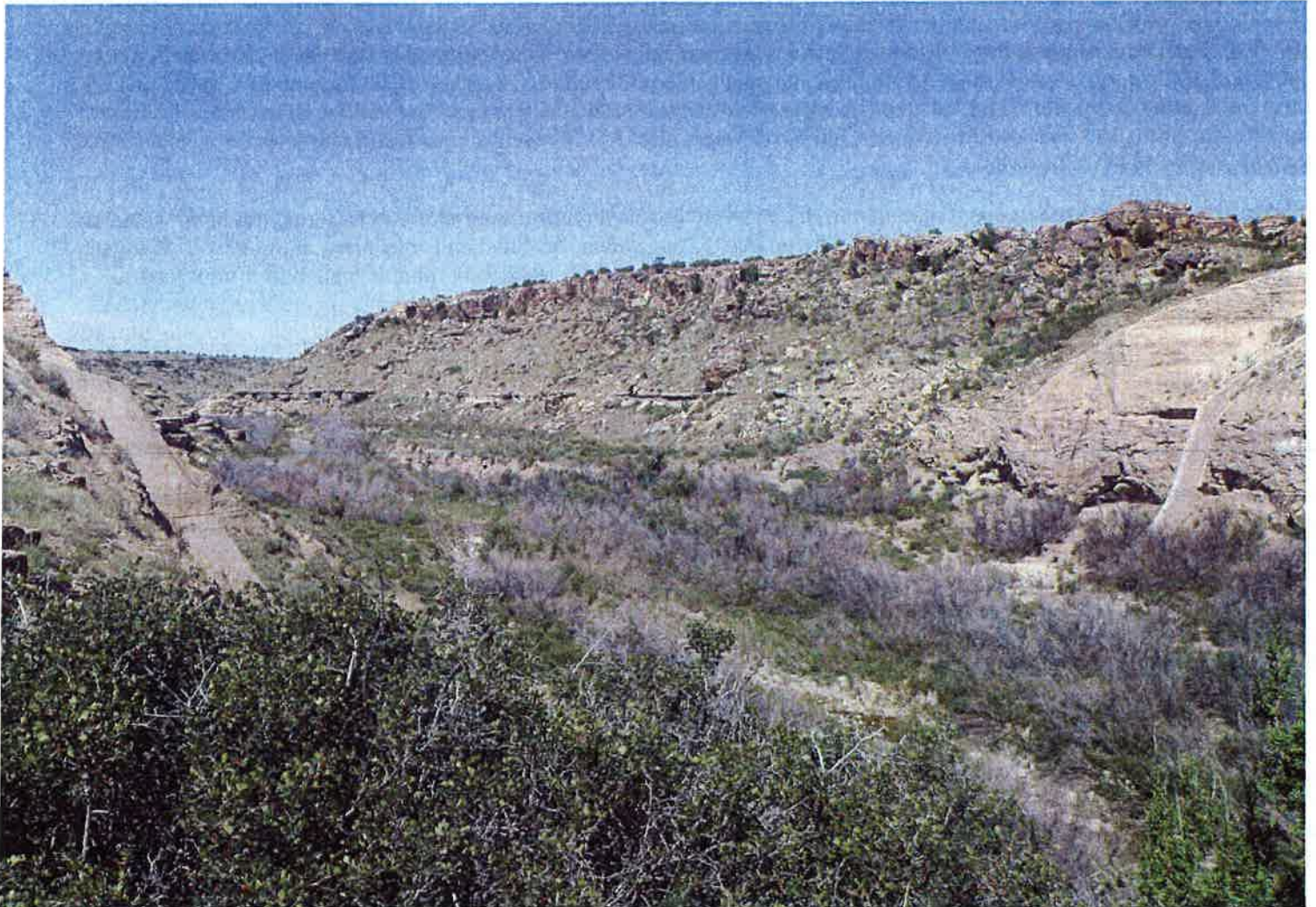
5LA.11666 Remains of the Apishapa Dam
