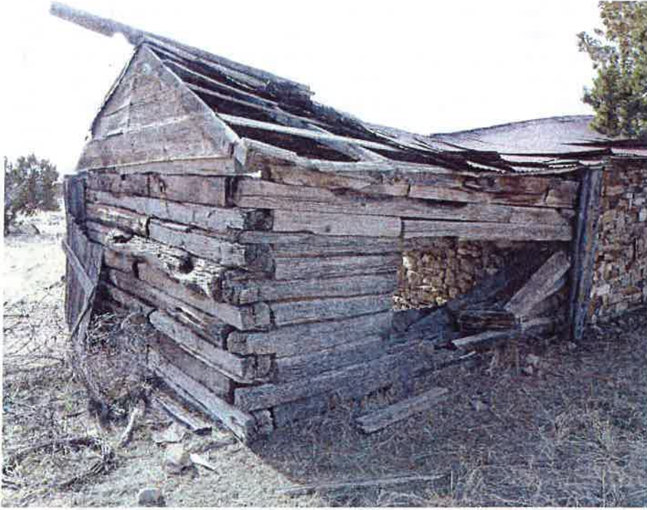
50T.1172 Barn constructed with stone and railroad ties
