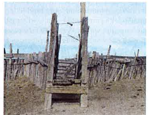
5LA.11897 Loading ramp
