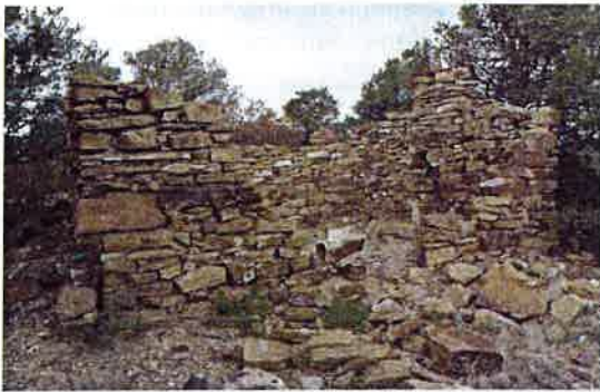
5LA.11840 Building of mostly fieldstone
