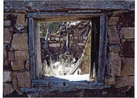
5LA.11781 Window frame of milled lumber
