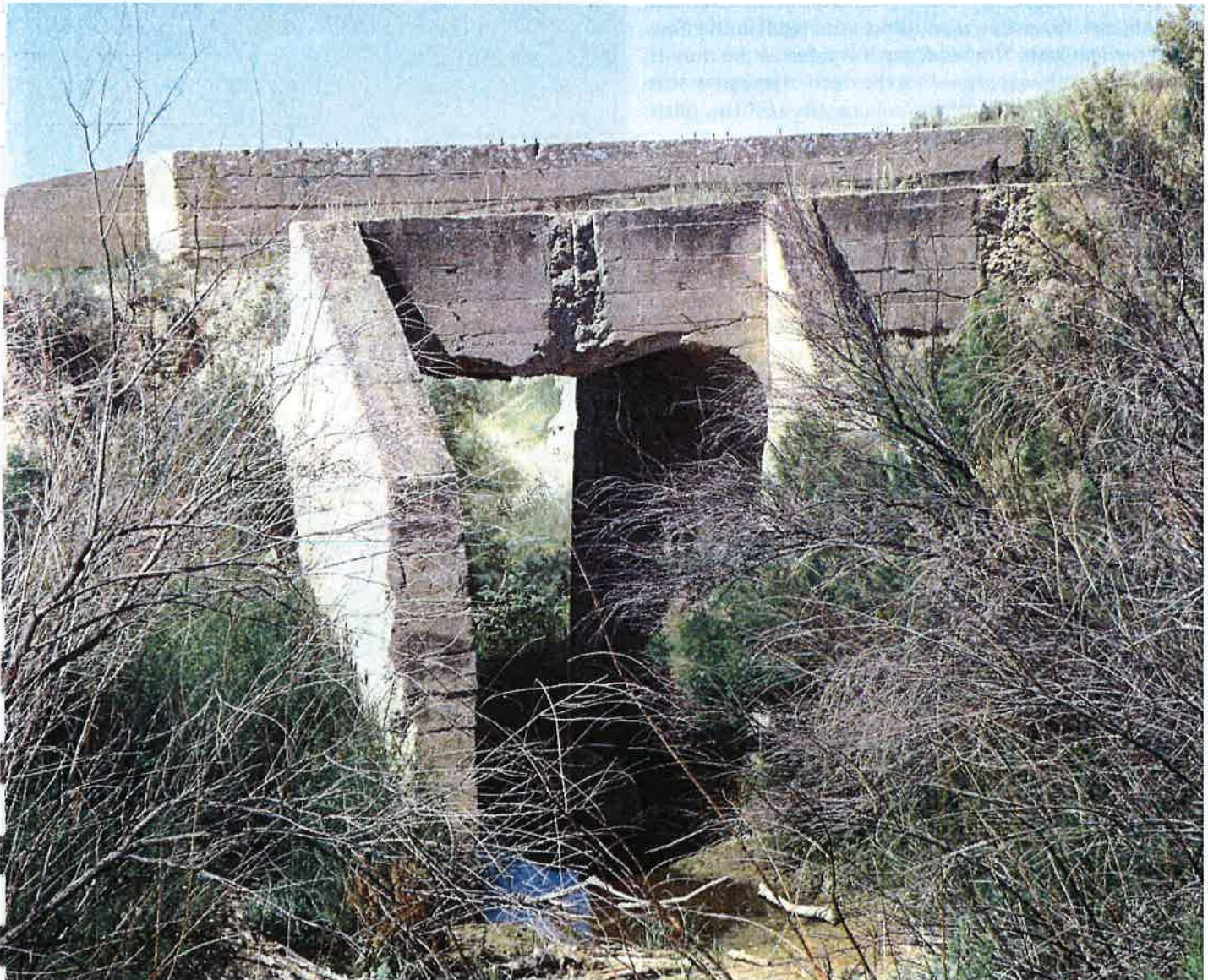
50T.1120 Part of the Timpas Creek diversion structure
