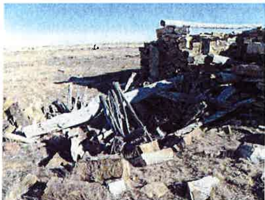
5LA.11853 Dugout with later addition
