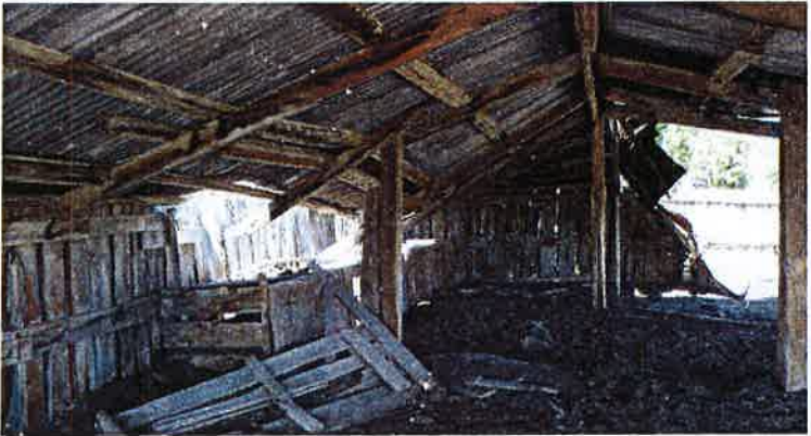
5LA.11717. Lambing shed
