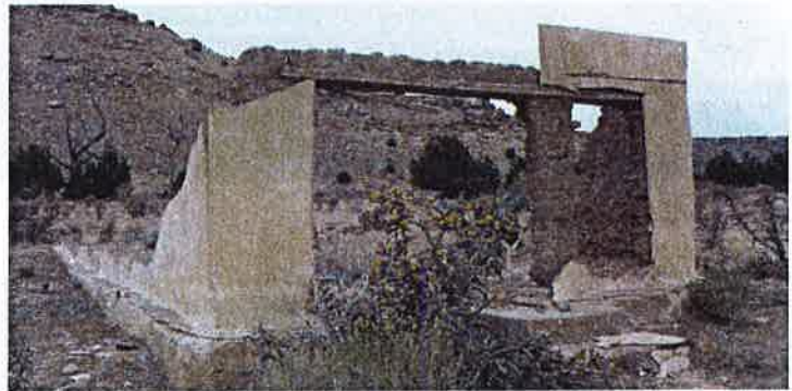
5OT.1177 Many of the region's schools also featured adobe block construction, such as the Higbee School
