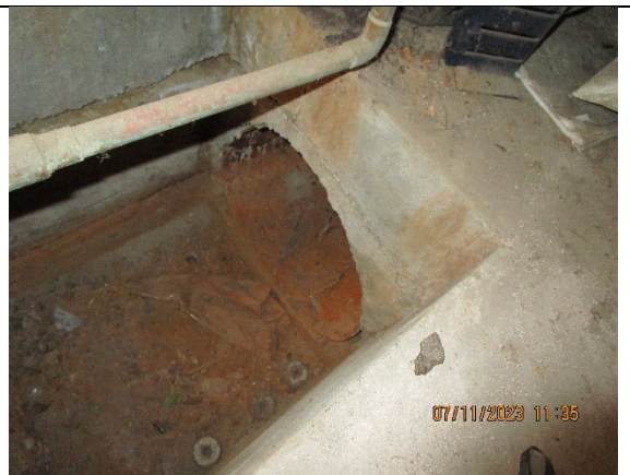
HVAC- Home Run
