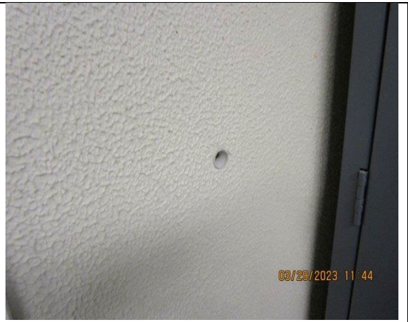
Rough Texture Drywall
